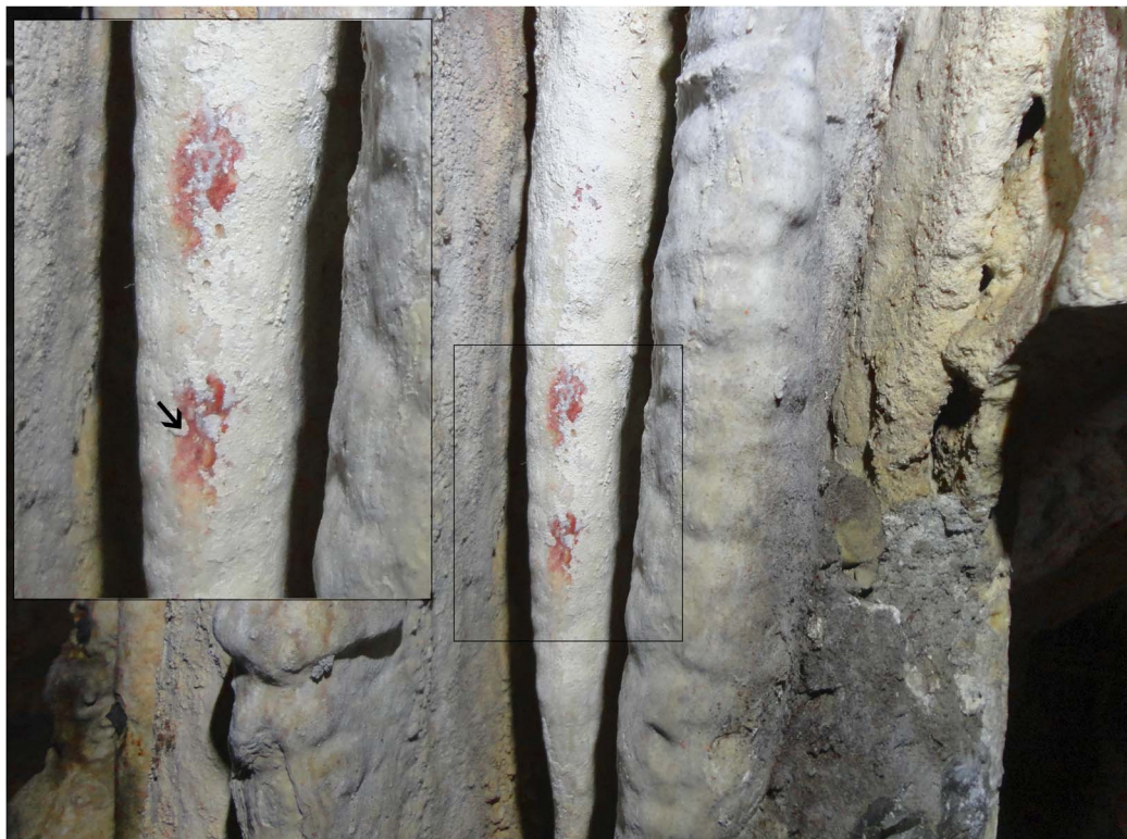
Figure 2 Picture of mark 1 with localization of the sampled point (GN14-17), in the area of the Balcon de Cascada en galerias Bajas .
